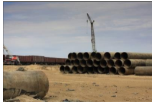
Gas pipes and freight carriages, Jaslyk
